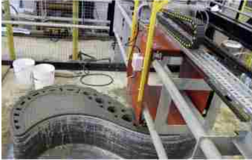
Figure 7: The Concrete Printing Process (Lim et. al., 2012)
